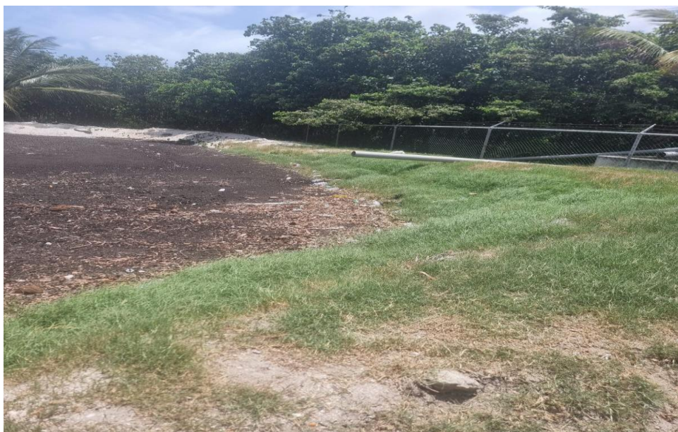
Photograph 9: WWTP Drying beds
