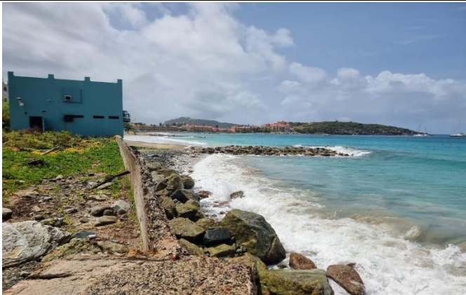
Photograph 7: Divi Little Bay – Opposite Green Building by the rocks
