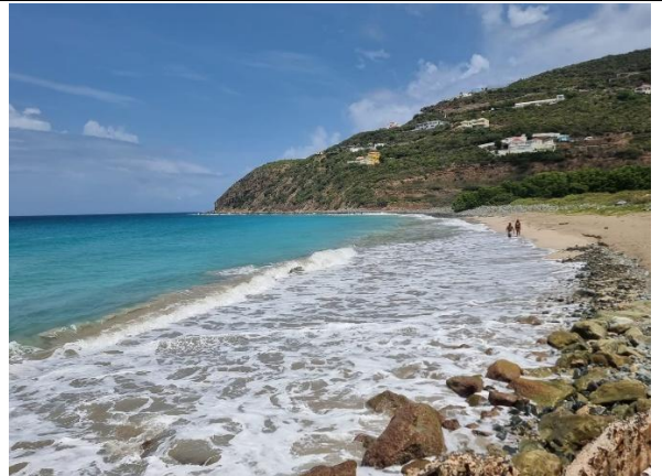
Photograph 8: DIVI Little Bay – Old Concrete staircase
