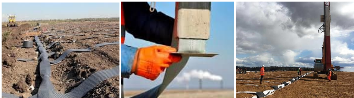
Figure 3.12 Visualization of installation of dense grid flexible landfill gas extraction system
